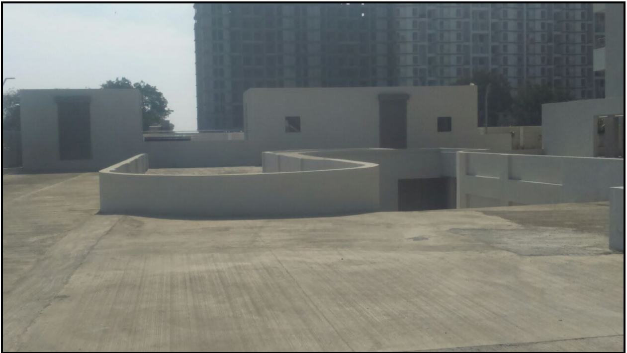
STP Pump Room
